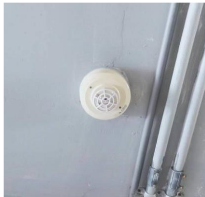
Heat Detector , Smoke Detector
