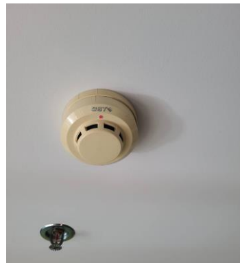
Heat Detector , Smoke Detector
